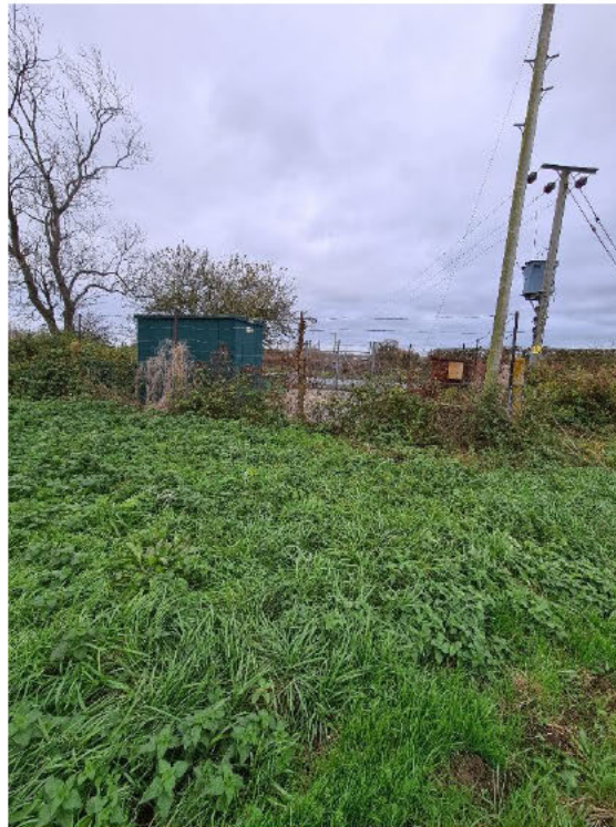
Picture Taken: 30/11/2021 Plate No. 18 Title: Substation located adjacent to the northern fields.
